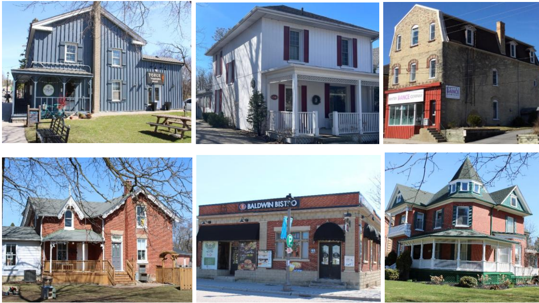
Photo 1 Roof shapes in the HCD from top left to bottom right: gable, hip, gambrel, cross gable, flat, and irregular
