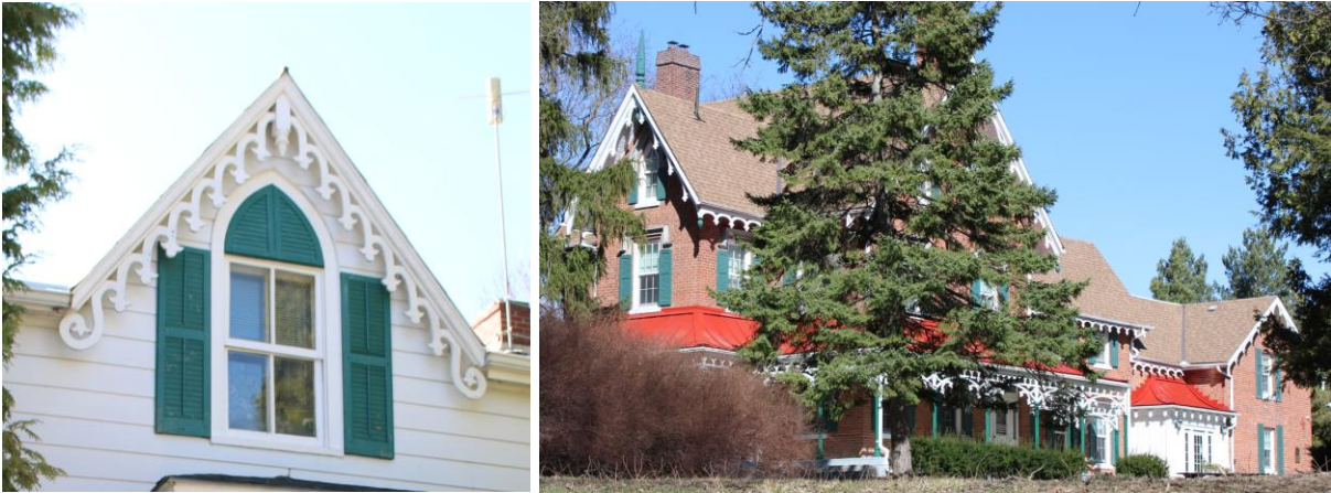
Photo 7 Examples of historic bargeboard in the HCD
