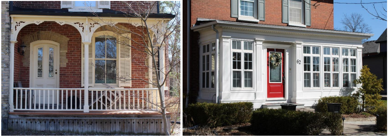
Photo 16 Historic porch examples in the HCD, including a covered partial wood porch, and an enclosed wood porch
