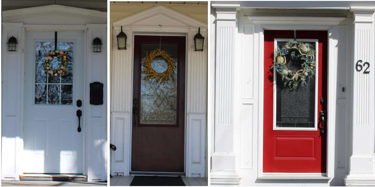
Photo 9 Examples of historic wood surrounds in the HCD, including dentils, pilasters, and panelling
