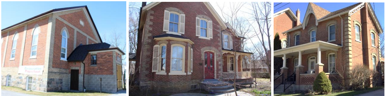
Photo 5 Examples of historic red brick with buff brick detailing in the HCD
