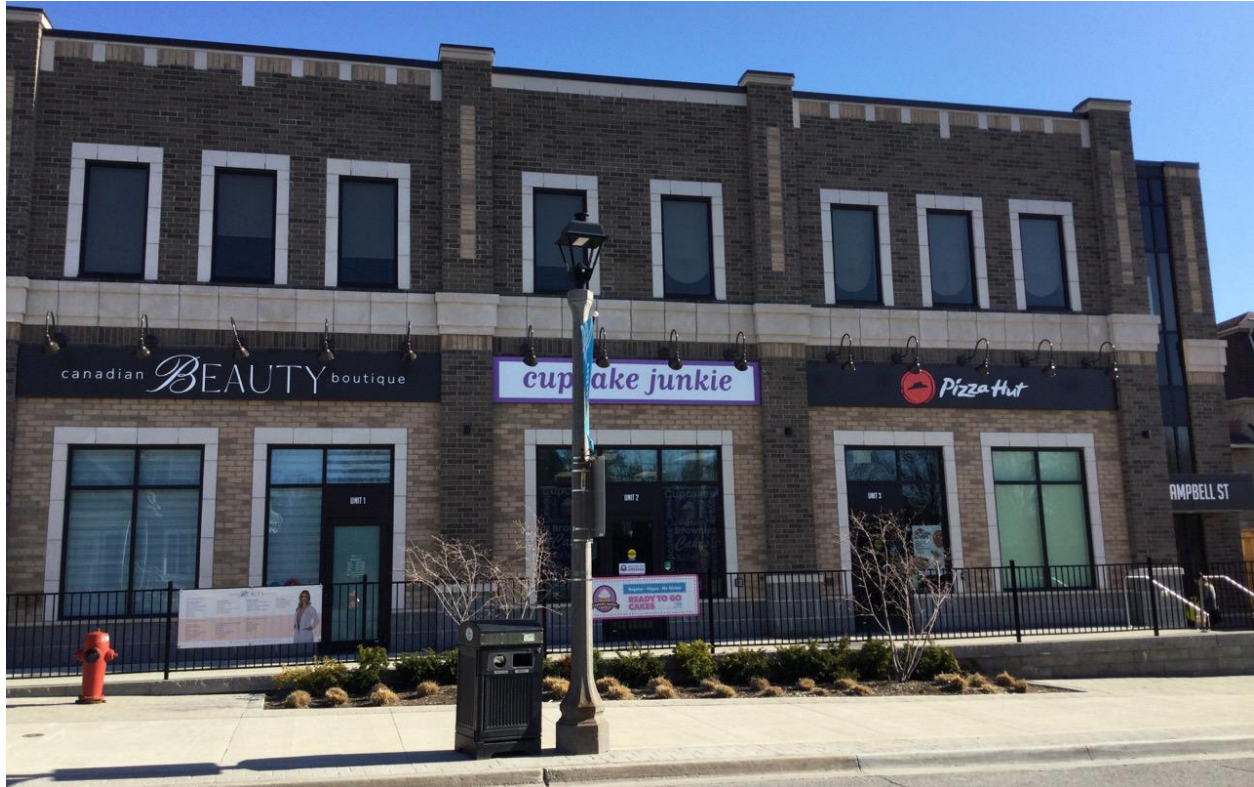
Photo 22 Appropriate new development in the HCD with vertical bays separated by a masonry course and pilasters with differentiating materials
