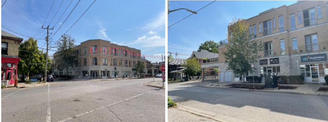
Photo 24 Examples of compatible medium density mixed use development that use brick and stone cladding, have regular fenestration patterns, and provide transitions to adjacent low rise buildings
