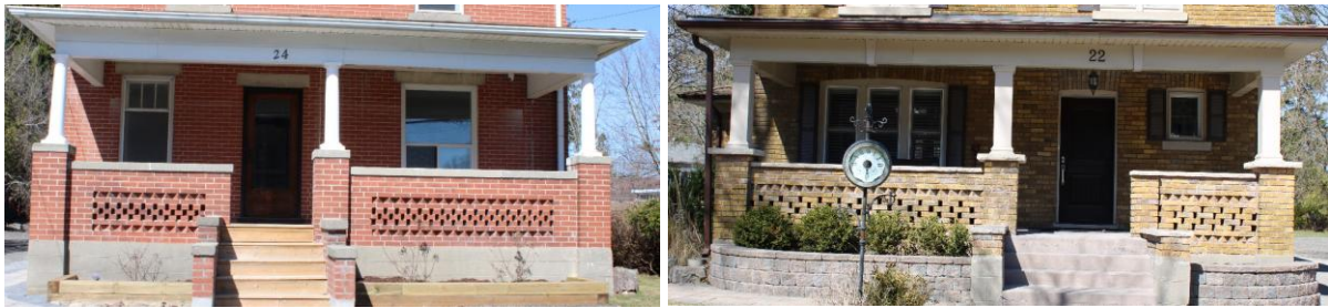
Photo 17 Two examples of covered brick porches with brick latticework in the HCD
