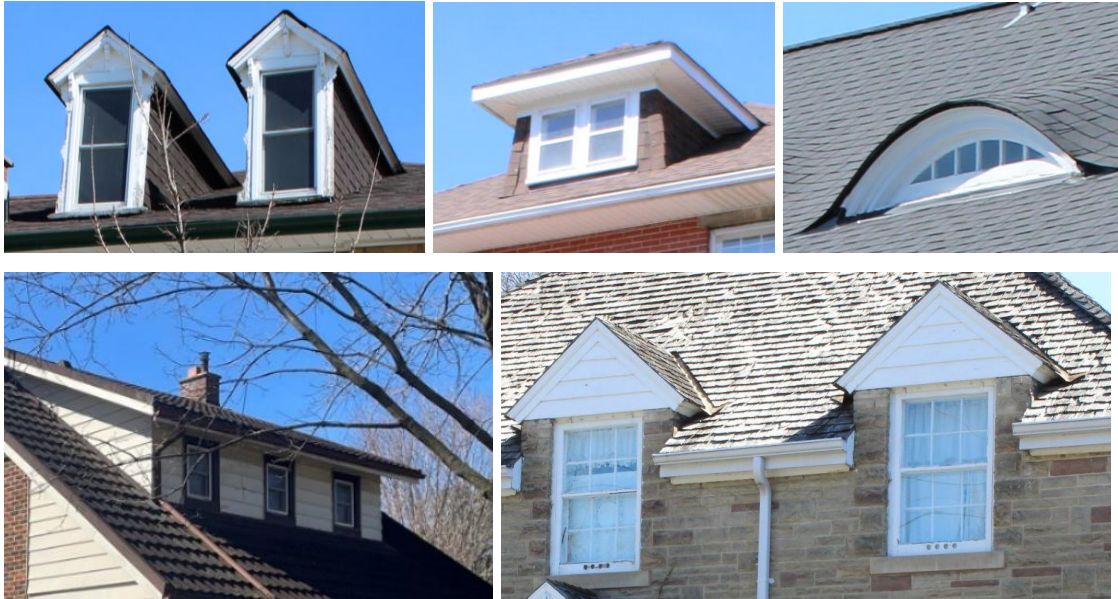
Photo 2 Examples of dormers within the HCD, including from top left to bottom right: gable, hip, eyebrow, shed, and wall gable
