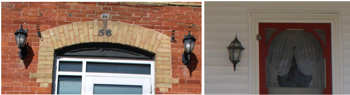
Photo 27 Examples of wall mount lighting in the HCD
