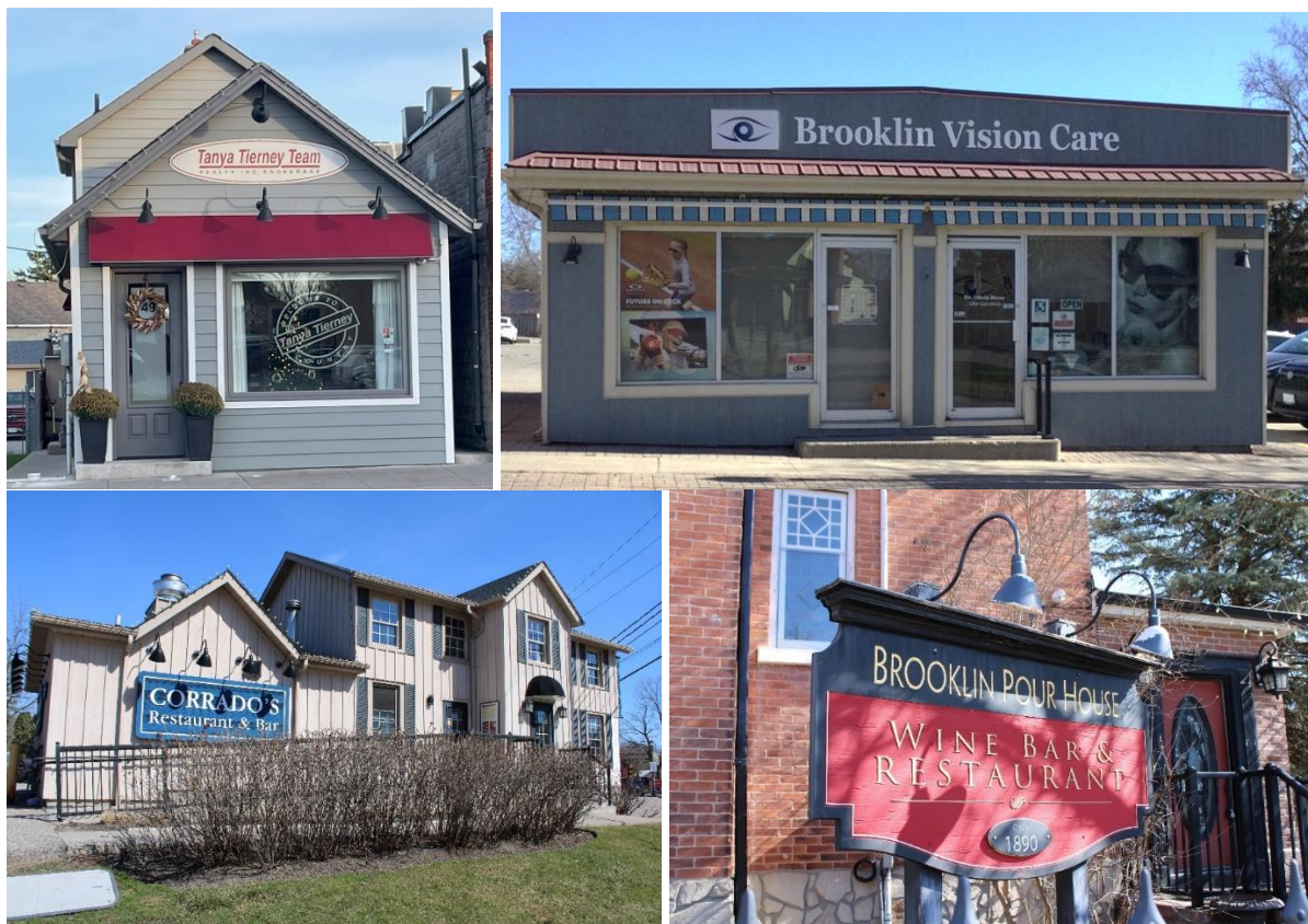
Photo 25 Examples of appropriate signage in the HCD
