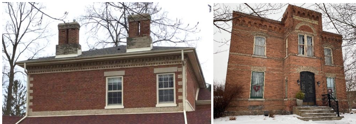
Photo 5 Examples of decorative brickwork in the HCD including dentils, voussoirs, quoins, and horizontal banding
