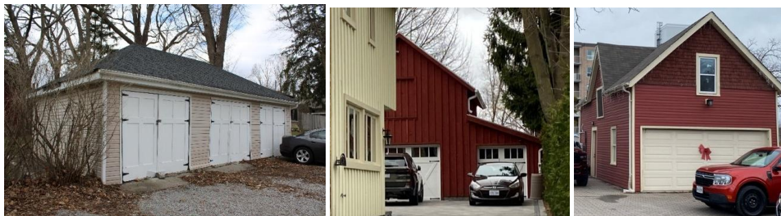
Photo 18 Examples of historic frame outbuildings in the HCD
