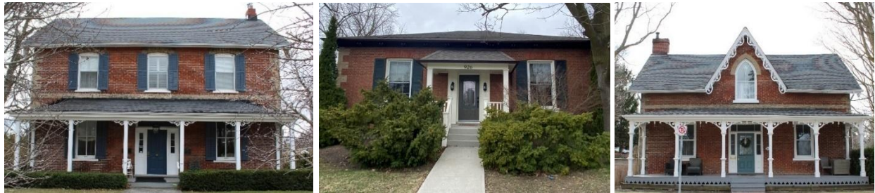
Photo 3 Examples of retained historic façade patterns including three bay façades with symmetrically placed windows, central doors and entrances
