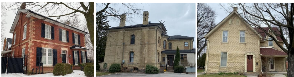
Photo 4 Examples of historic brick masonry in the HCD including red brick, buff brick, and one unique residence with brick frogging
