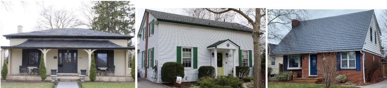
Photo 2 Low, medium, to high pitch roof examples in the HCD, including hip and gable roofs
