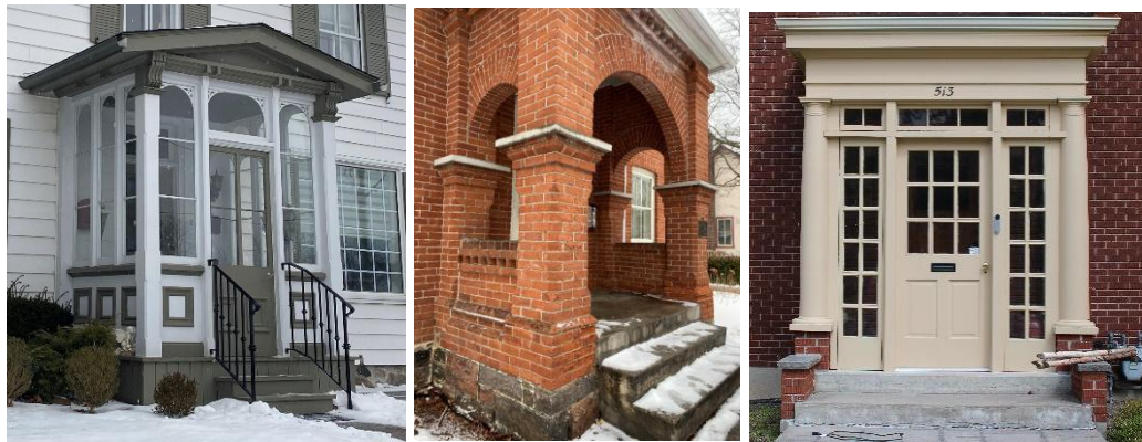
Photo 16 Examples of historic entrances within the HCD
