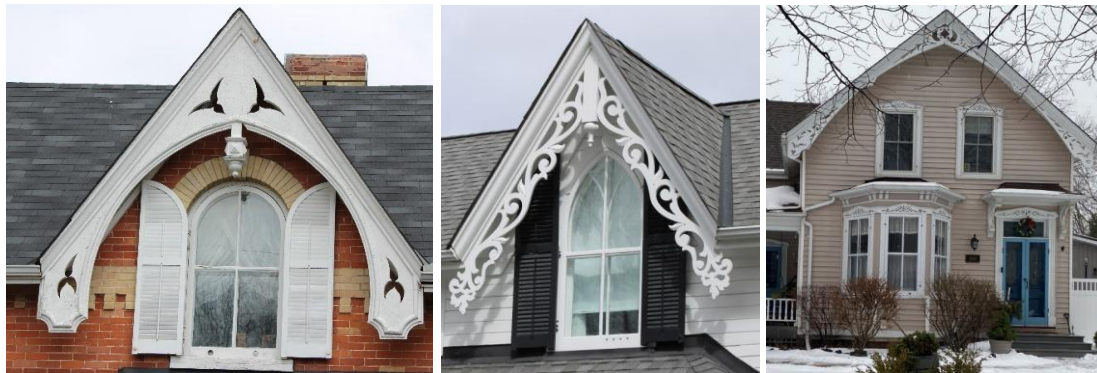
Photo 8 Examples of woodwork in the HCD including bargeboard, shutters, sills, storm windows, and window and door surrounds.
