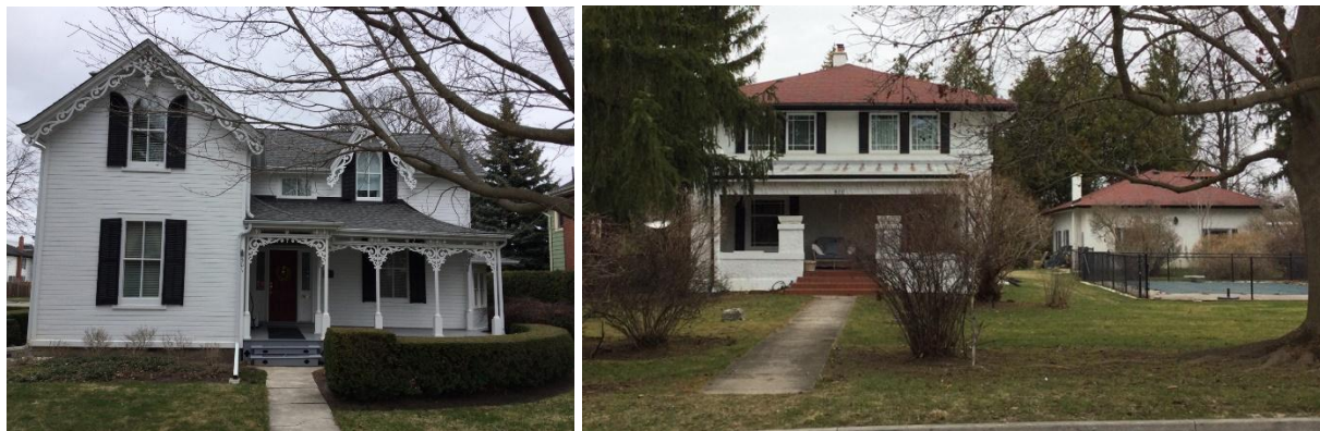
Photo 7 Examples of historic wood clapboard (left) and stucco (right) in the HCD
