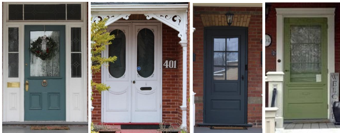
Photo 13 Examples of historic entrances within the HCD
