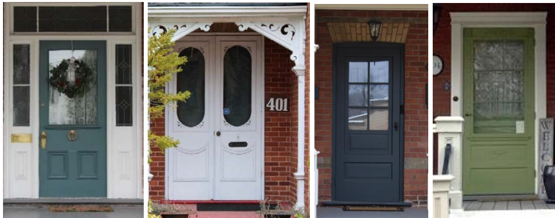
Photo 13 Examples of historic entrances within the HCD
