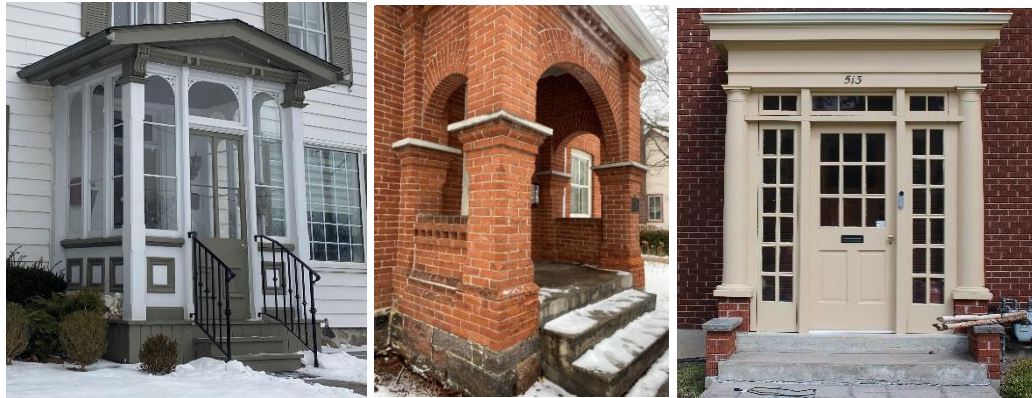
Photo 15 Examples of historic entrances within the HCD
