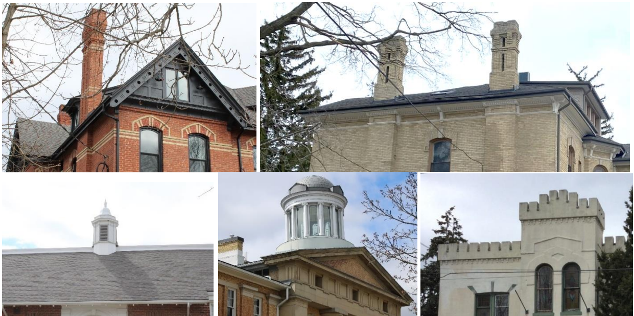
Photo 1 Examples of character defining roof features in the HCD including brick chimneys, eaves, cupolas, and parapet battlements
