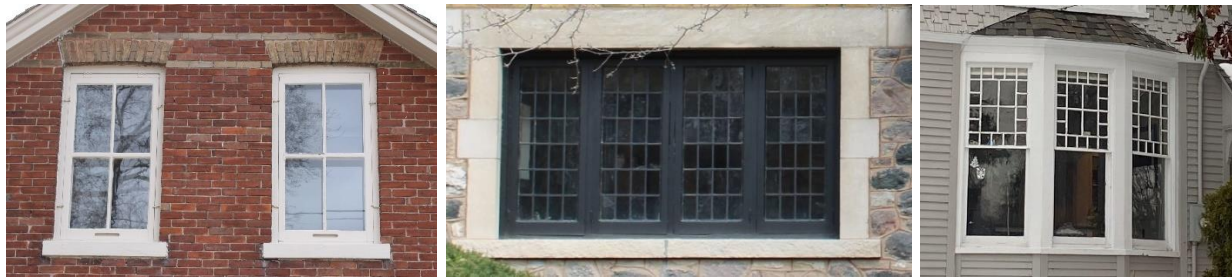
Photo 11 Examples of historic windows in the HCD including 2/2 wood sash, multi-pane casement, and bay windows
