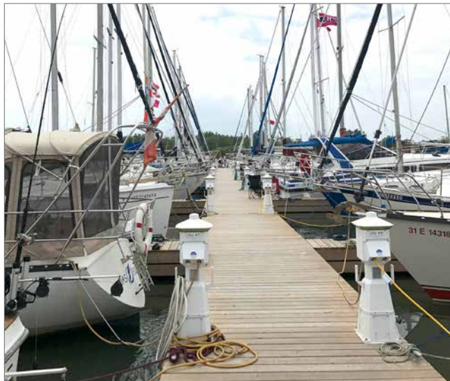
Port Whitby Marina pier
