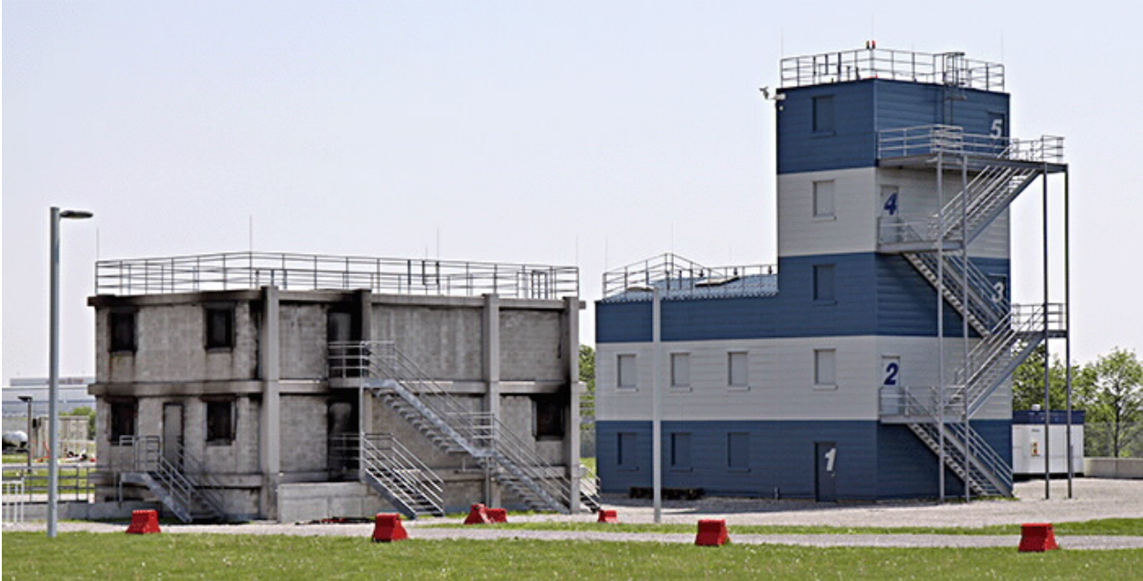
13.12 Figure 96 – GTA Training Towers
