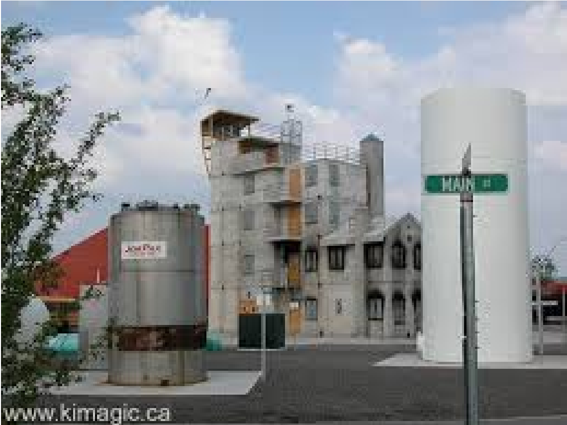
13.13 Figure 97 – Oakville Fire Training Facility
