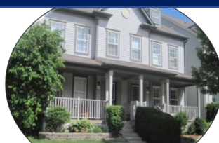
Two units attached by a common vertical wall.
