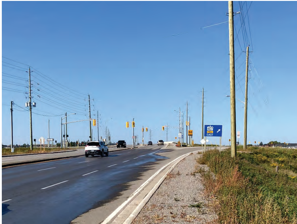
Photo 3: Highway 407 East Interchange North of the Study Area
