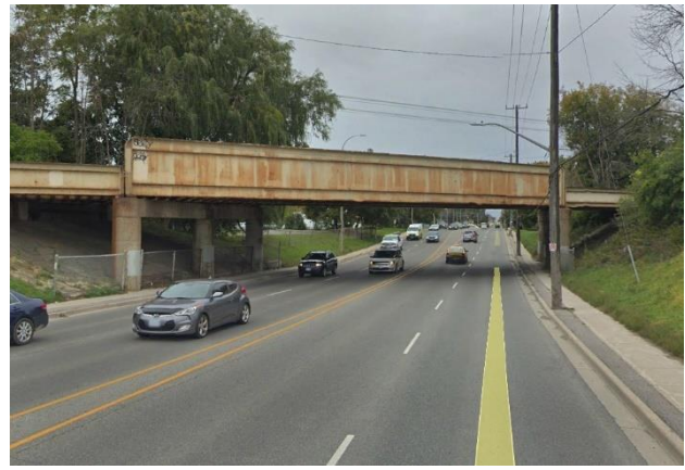
Photograph 4: Bridge BR_D07_04 at Dundas Street East
