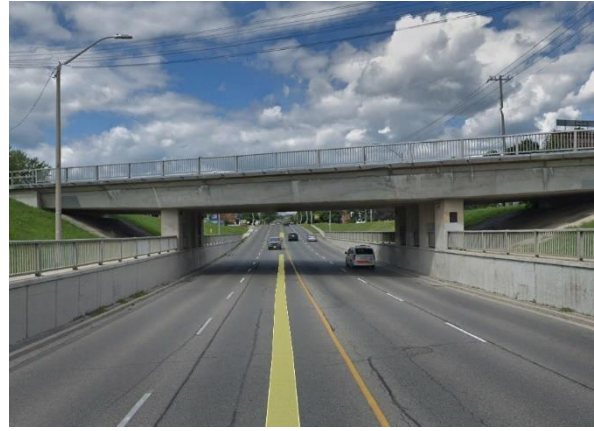
Photograph 2: Bridge BR_C04_03 at Brock Street North
