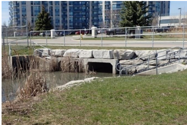
Photograph 5: Culvert CU_D01_03 outlet
