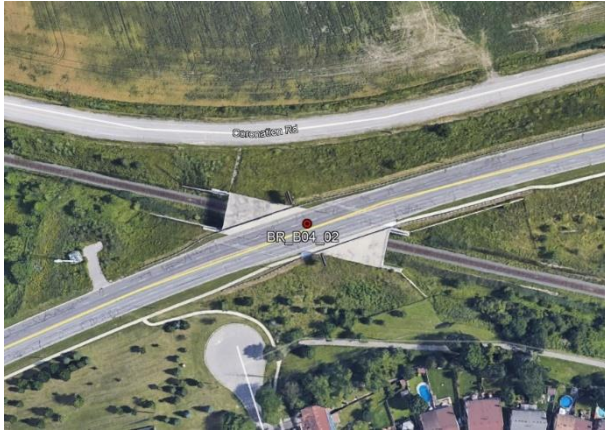
Photograph 1: Bridge BR_B04_02 at Rossland Road West
