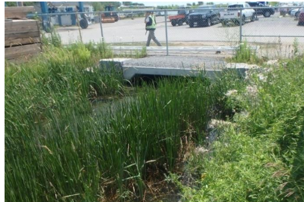
Photograph 6: Front Street West Culvert Inlet during Low Flow Conditions
