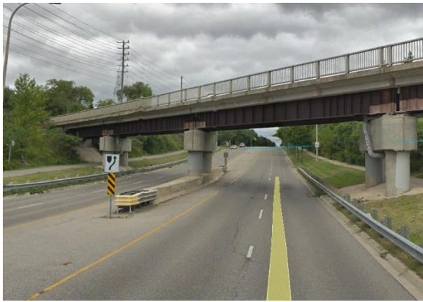
Photograph 3: Bridge BR_C04_04 at Garden Street
