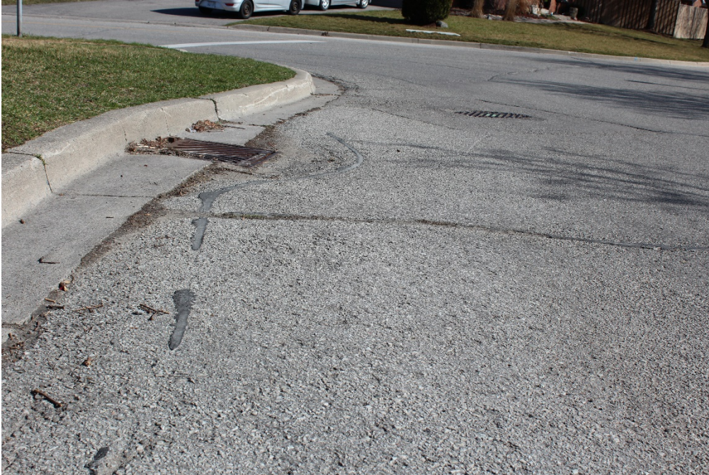
Figure 12 A photo of a road in Fair condition
