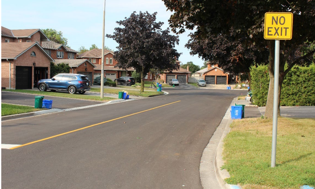
Figure 10 A photo of a road in Very Good condition
