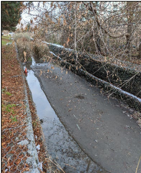
Sediment accumulation in channel between Victoria Street West and Watson Street West
