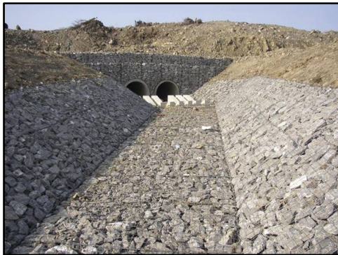
Example of Gabion Mattress
