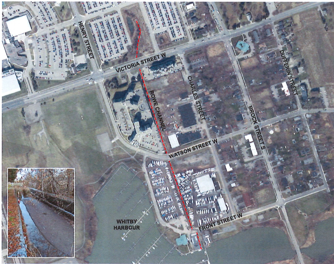
Figure 1: Location of the Rowe Channel (dashed red line) in the Town of Whitby. Inset shows the concrete and gabion-basket lined channel north of Watson Street W. All site disturbance/alteration will be limited to the Rowe Channel itself.
