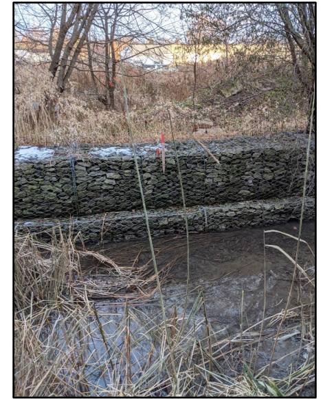
Gabion Baskets within Rowe Channel
