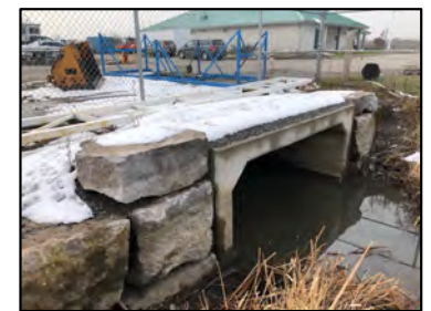
Front Street W Culvert
