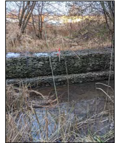
Gabion Baskets within Rowe Channel
