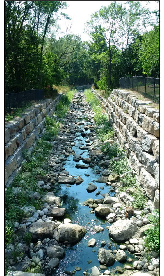
Channel with Armour Stone Example Note this site is larger than Rowe Channel
