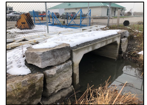
Front Street W Culvert
